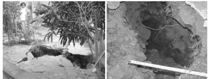
Fig. 24 Cracks and soil displaced in the Villa de Álvarez sand liquefaction event.
