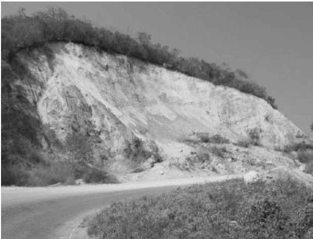
Fig. 26 Landslide in the Colioma-Tecomán highway (100,000 m 3 )
