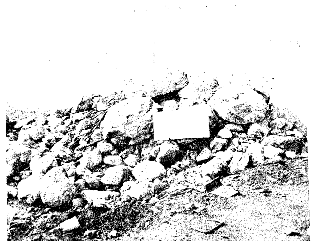
Fig. 4 - Material hauled off the stilling basin by divers.
