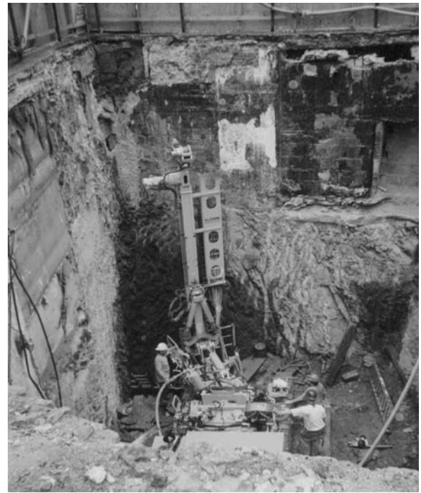
Fig. 12. Drilling corner caissons adjacent to NYCT structures
