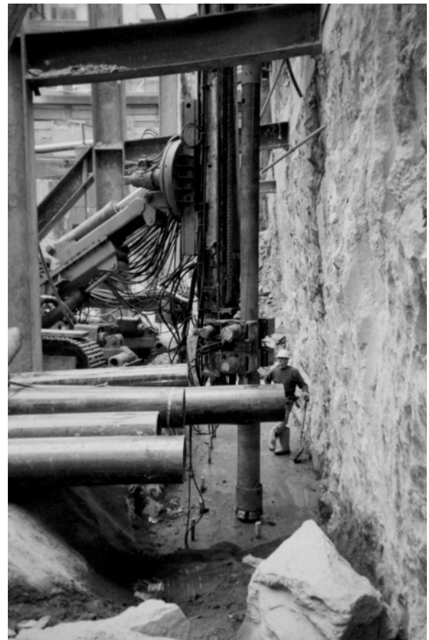
Fig. 9. Caisson installation at 5 Times Square adjacent to NYCT subway structure
