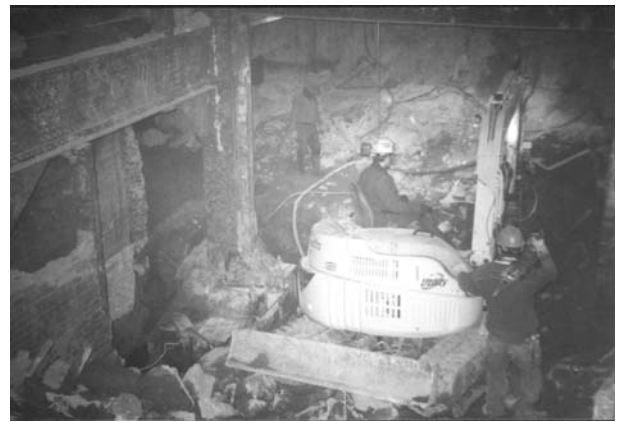
Fig. 15. Excavating with small equipment around existing foundations below active subway station
