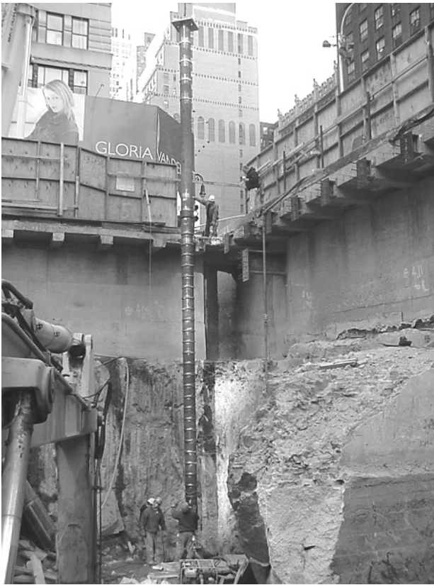
Fig. 14. Installing 13-inch diameter core in column caisson
