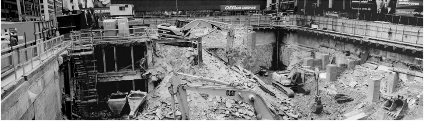
Fig. 11. 7 Times Square site, looking south during foundation construction
