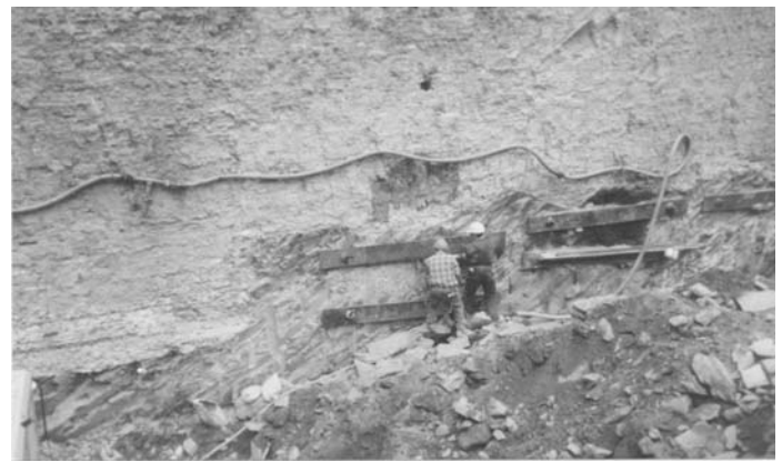
Fig. 8. Rock bolting below the New Amsterdam Theatre
