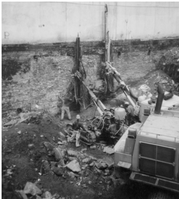
Fig. 7. Channel drilling adjacent to the New Amsterdam Theatre
