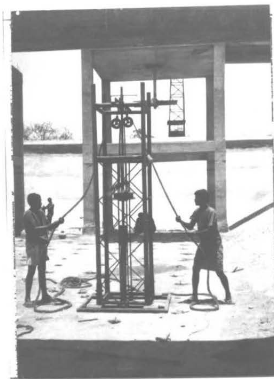
Fig. 7 Photograph of the arrangement for sand piling.
