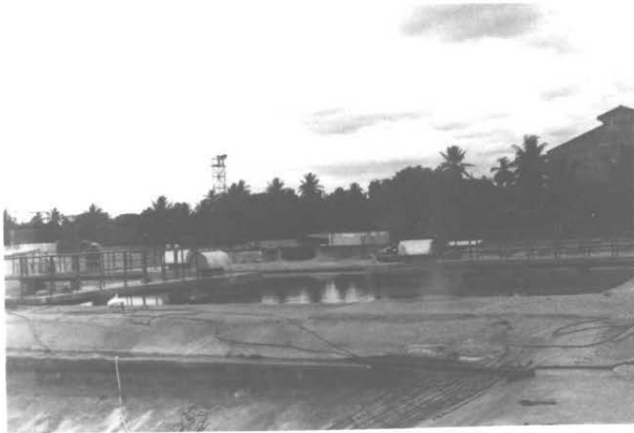
Fig. 9 Photograph of the restored equalization tank after commissioning into operation.
