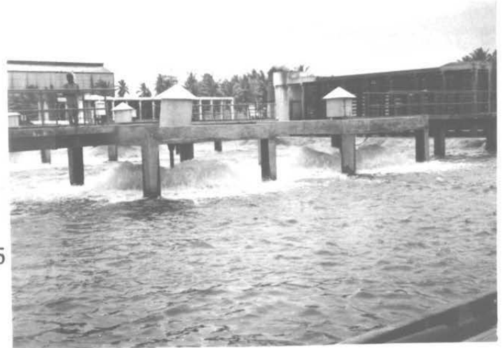
Fig. 10 Photograph of the restored aeration tank after commissioning into operation.
