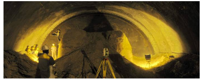
Fig 4 NATM excavation method in T4 section
