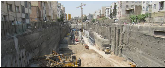
Fig 5 Cut & Cover method in T2 section
