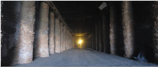
Fig 6 Top/Down method in T4 section
