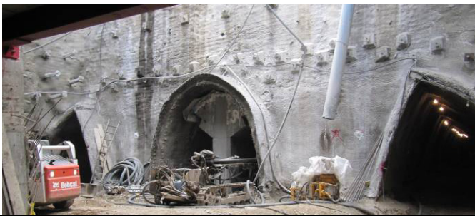
Fig 7 Nailing at TU Portal area
