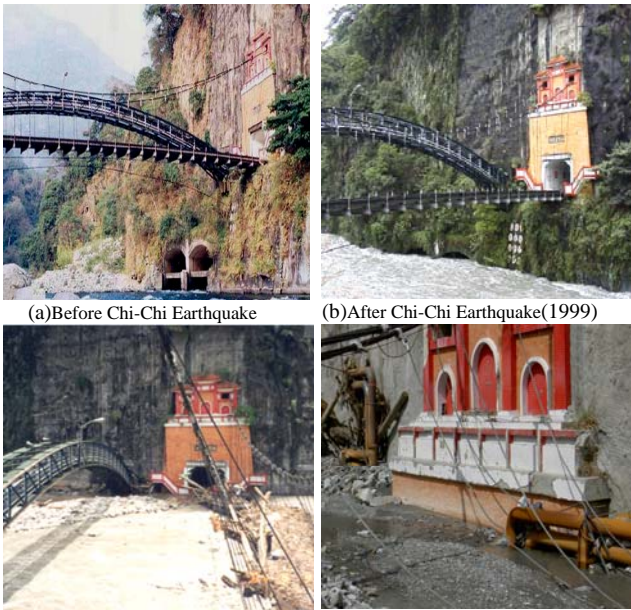
(a) Before Chi-Chi Earthquake (b) After Chi-Chi Earthquake(1999) (c) After Toraji Typhoon(2001) (d) After Mindulle Typhoon(2004) Fig.7. Riverbed changes in front of Kukuan power house after the disastrous events
