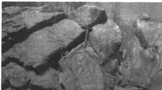
Fig.2 : Open-jointed rock with dislodged blocks in North Koel dam foundation.
