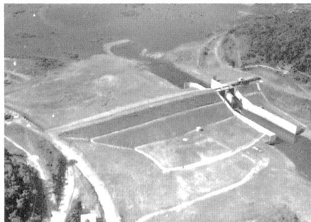
Fig. 1. The Santa Helena Dam
