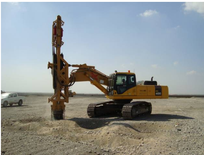
Photo 2. Soil Improvement Operations via Rapid Impact Compaction (RIC).
