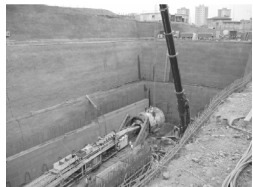
Fig. 18. Soil Nail Retaining Wall
