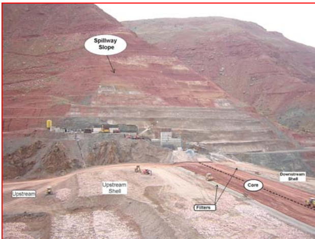
Fig. 6. A view of the slope and Dam body (front view)
