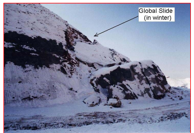
Fig. 8. Global slide occurred in the slope
