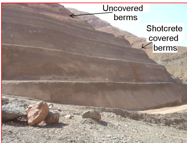
Fig. 7. A view of the slope (side view)
