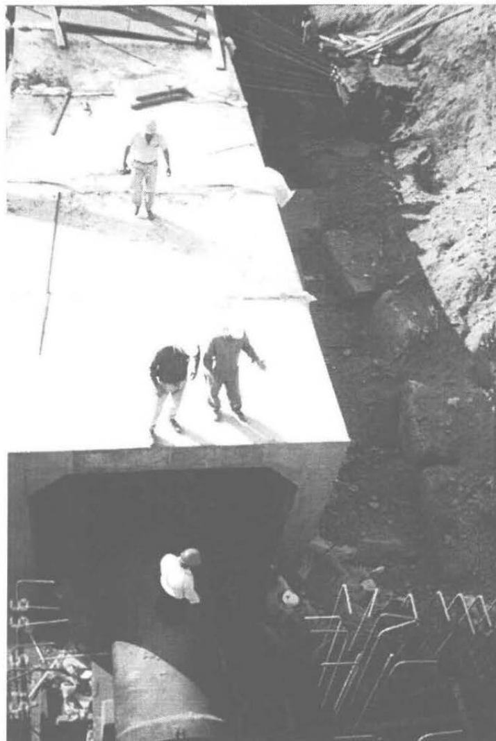
Fig. 8 Utilidor construction over 1.4-m diameter pipe.
