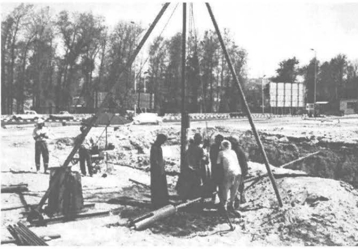
Fig. 5 Hand-auger bucket soil boring.
