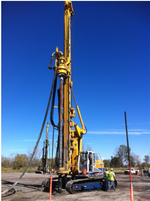
Figure 9: Installation of CMC's with Reinforcing Bar
