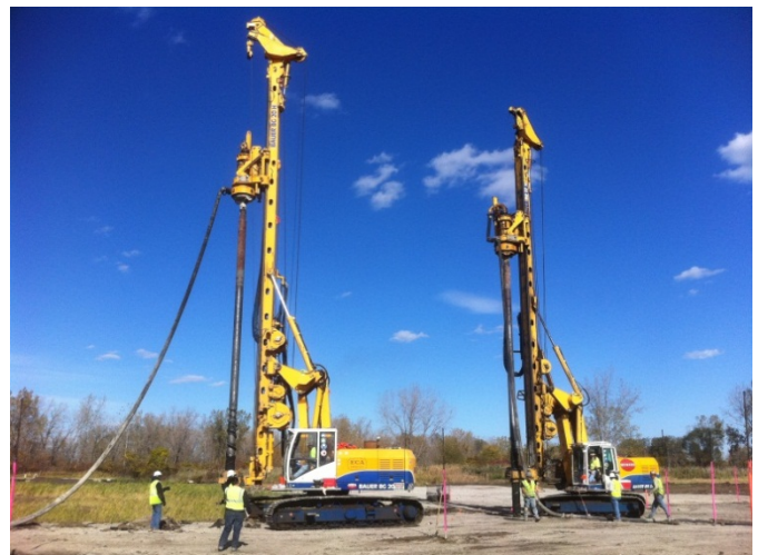
Figure 8: Installation of CMC's at Project Site
