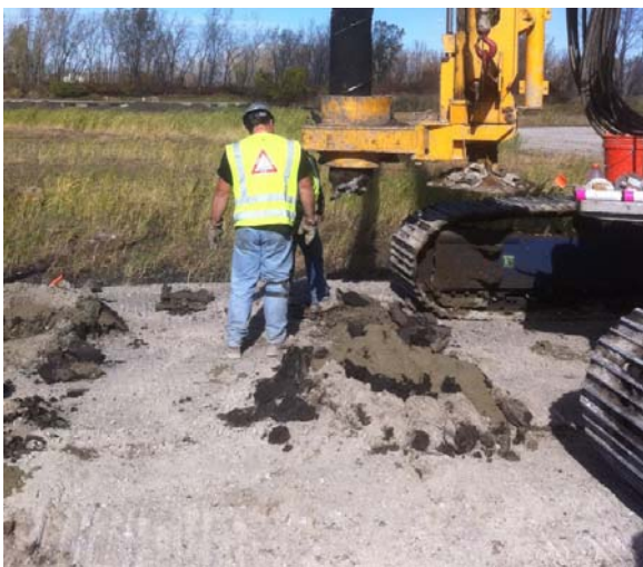
Figure 10: Minimal Soil Cuttings from Installation Process
