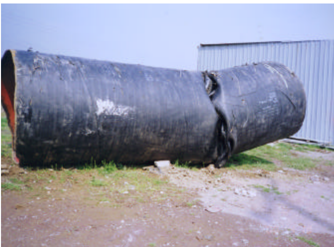
Fig.7. Highly deformed water pipe due to fault striking
