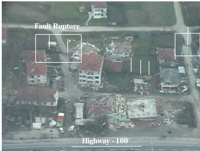
Fig.6. Collapsed and damaged residential buildings along Highway-100 due to fault surface rupture (modified from the USC-GEES web-site)
