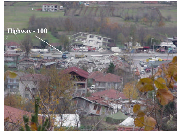
Fig.8. Heavily damaged central section of Kaynasli, (source: USC-GEES)
