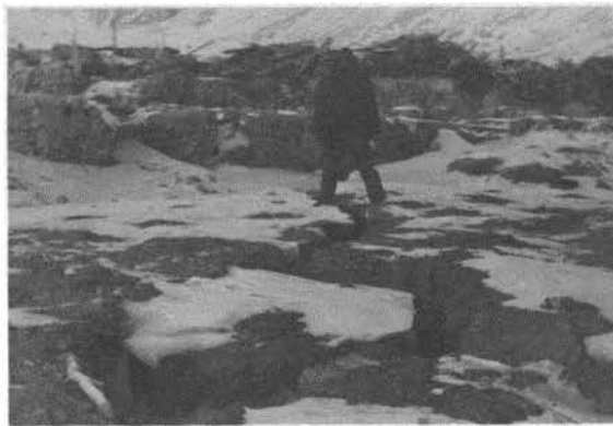
Fig. 5. Ground fissures which cut across Kaurik village.
