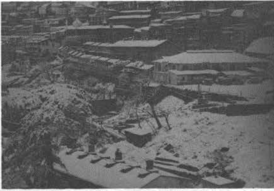
Fig. 4. Buildings constructed on stable ground in Kinnaur.
