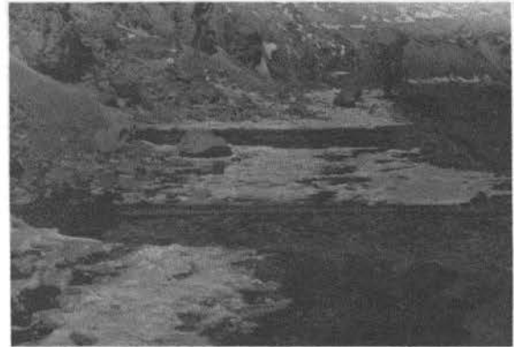
Fig. 7. Step faults across road between Sumdoh and Kaurik.
