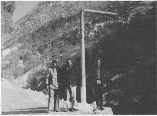
Fig. 14. Bending of telegraph pole resulting from impact of flying rock fragments.
