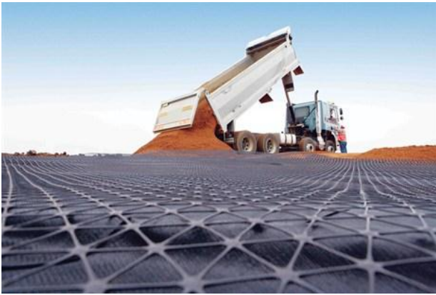
Fig. 21 Geosynthetics in Road Construction on Soft Soil
