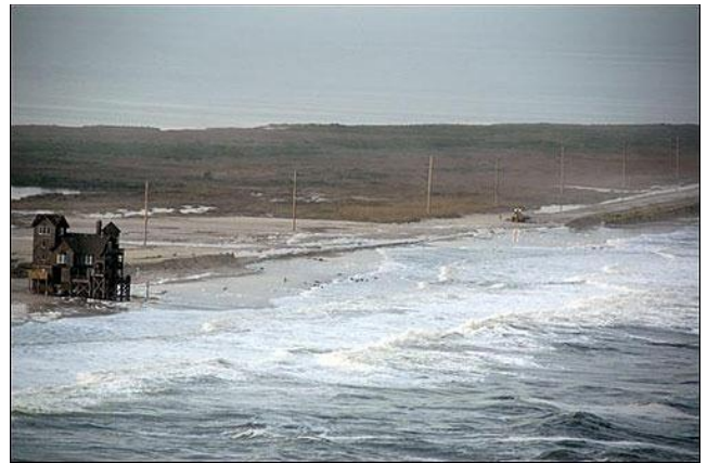
Fig. 6 North Carolina Coastal Highway 12 Overwash – 2006
