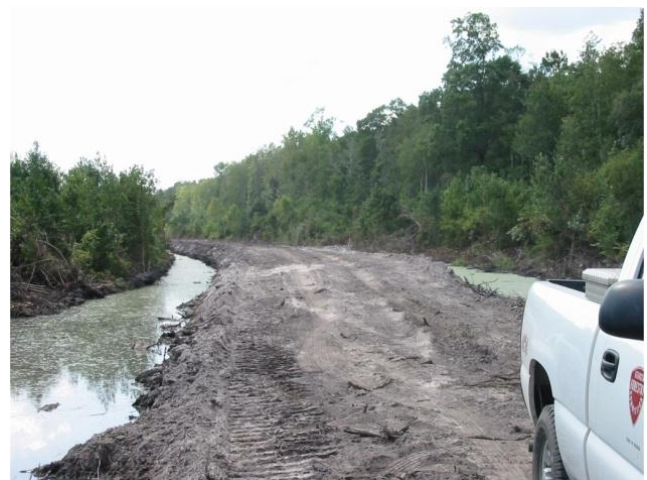
Fig. 16 Mile long road under construction through wetland
