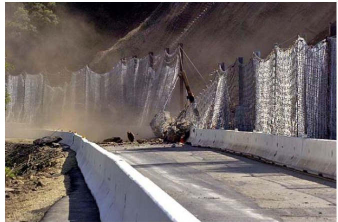
Fig. 12 2006 Rock-Slide - Highway 140 near Yosemite, CA
