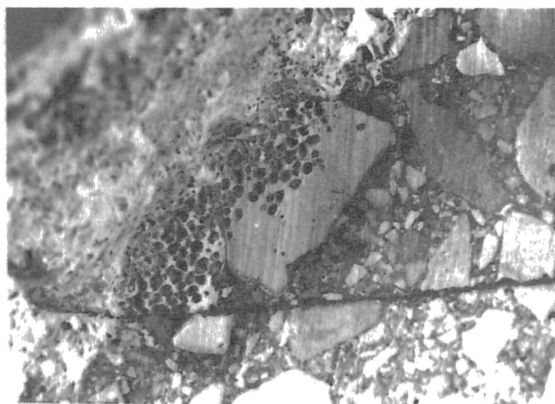
Figure 7 Sawcut Pile Section showing Sponge Infestation in Concrete Aggregate
