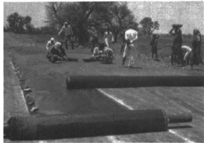
Fig.2 : Laying of Geotextile over Finished Subgrade
