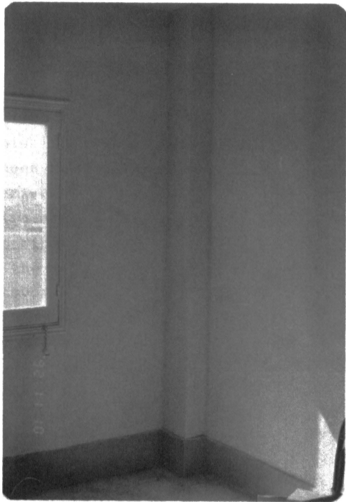
Photo 3 Same Column of Photo 2 in the Western Site Building
