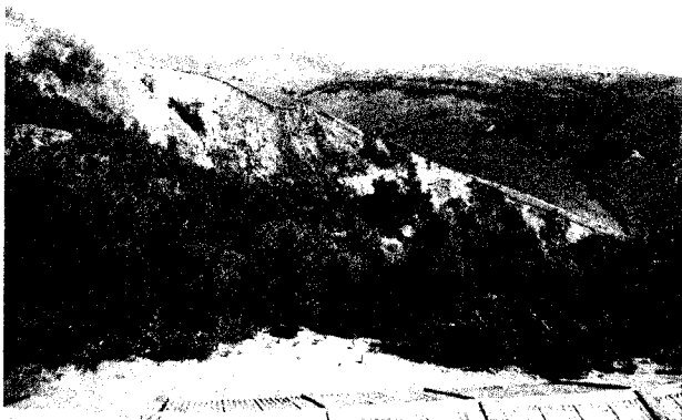
Fig.1 Panoramic View of the Landslide.
