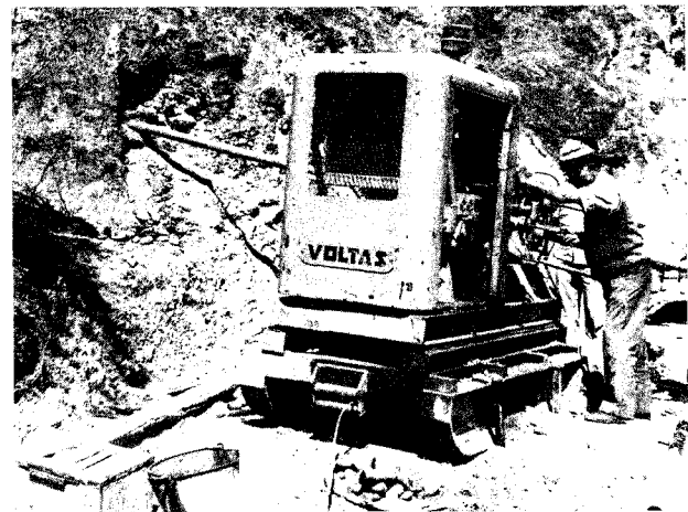
Fig.2 Drilling rig in operation
