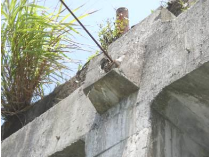
Fig. 9 (a) Tendon fracture and shoot out
