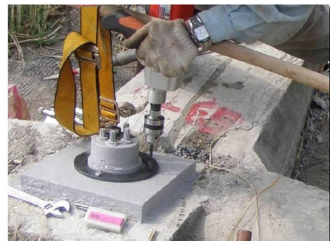
Fig. 16 (a) drilling screw hole on bearing plate
