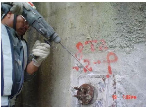
Fig. 15 (a) Drilling grout exit or air vent hole
