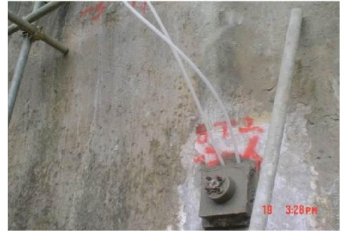
Fig. 15 (b) Setting grouting pipe and air vent pipe
