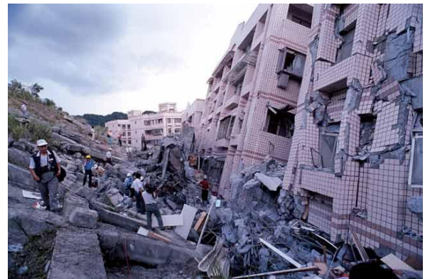
Fig. 8 Landslide of Lincoln Mansion in 1997
