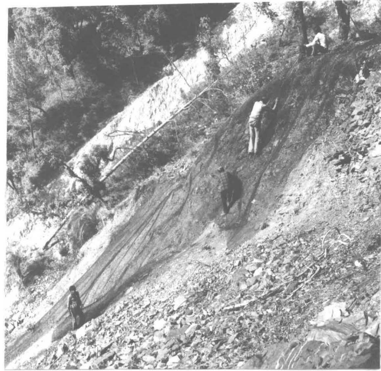
Fig.1 Fixing of the synthetic geogrid for rock fall control.
