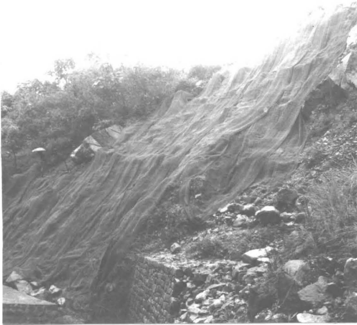
Fig.4. Slope treatment with coir netting.
