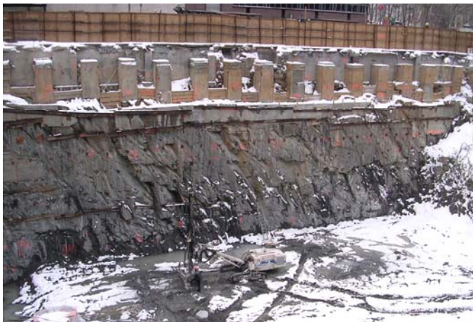
Fig. 17. 6th Avenue Rock Cut
