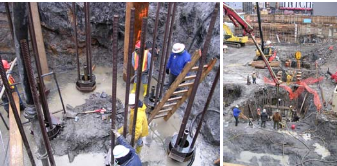
Fig. 7. Grouting of Caissons at NYT Tower
