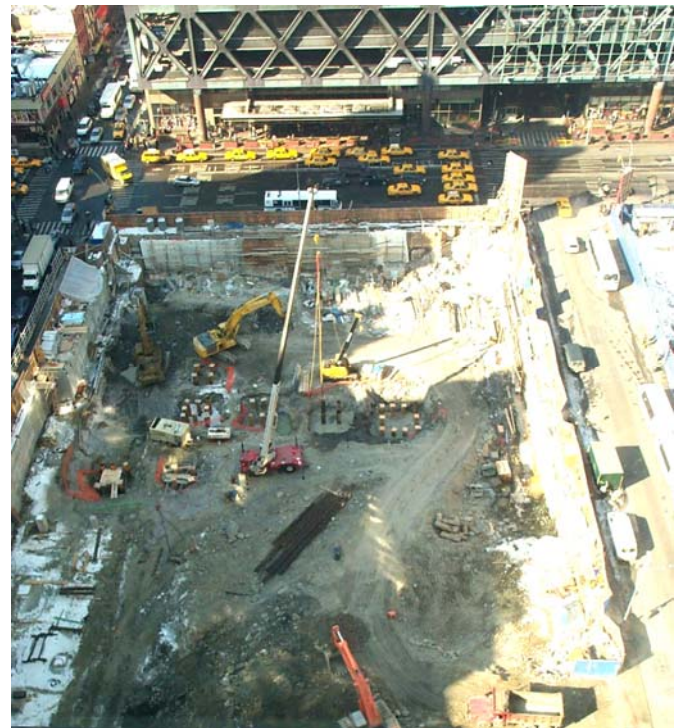
Fig. 8. Overhead View of Caisson Caps at NYT Tower
