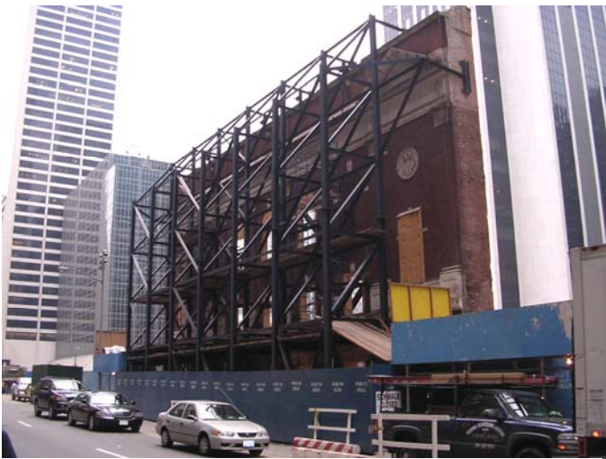
Fig. 19. Above Grade Theatre Façade Stabilization
