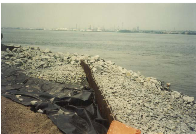
Fig. 14: Butress of Crushed Stone, Riprap and Geotextile
