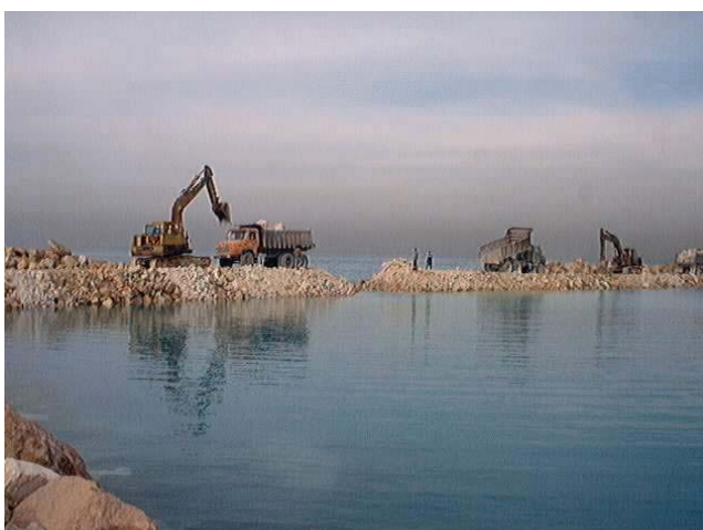
Fig. 2. A view of basin construction
