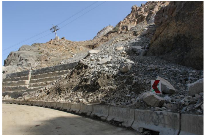
Fig. 5. Debris flows at a gully.
