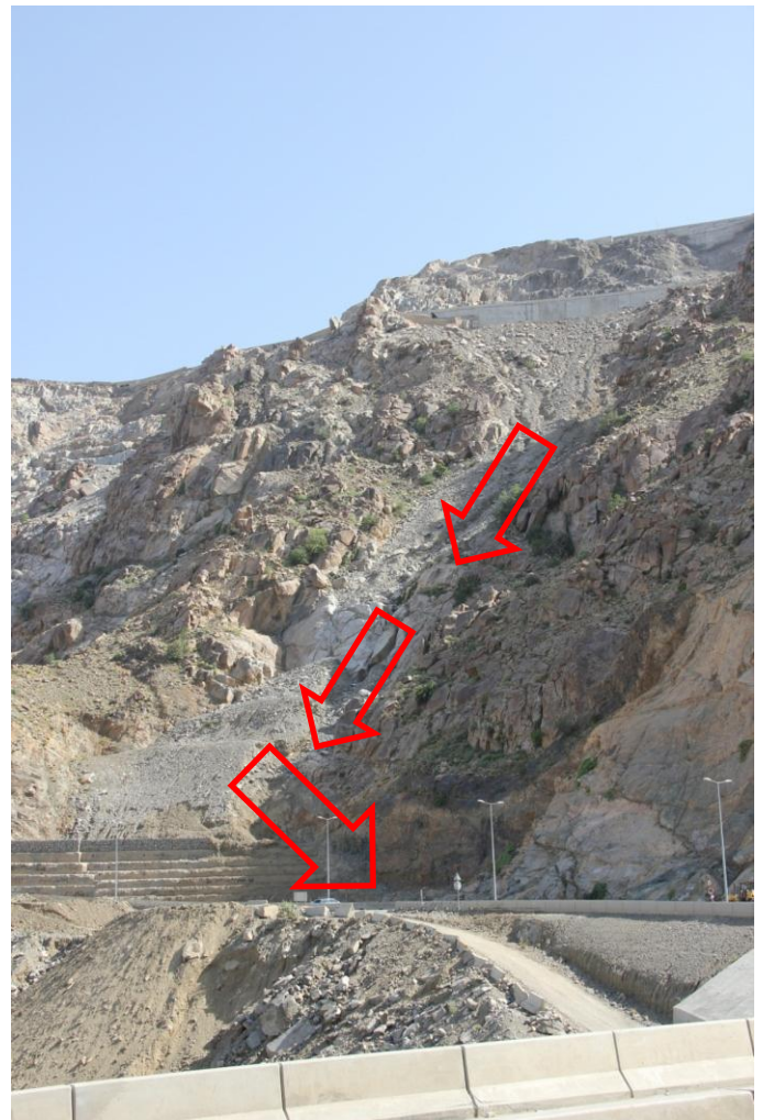
Fig. 7. Terraces at the debris engraved due to rainfalls, was not stabilized against the rainfall flow incision effects.
