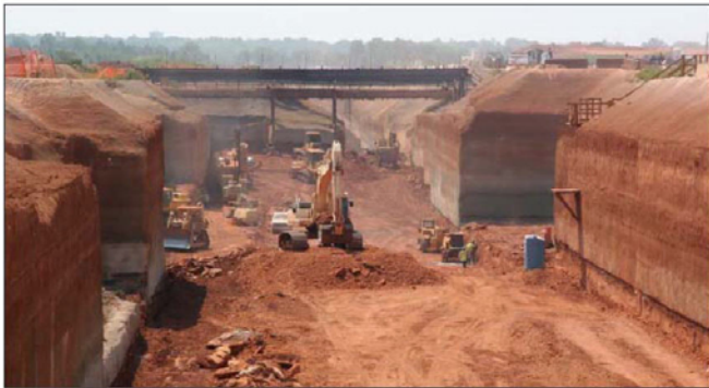
Figure 11: Typical rock cuts at Dulles Airport site (Tier 3 Excavation, photo from McQuinn et al 2006)
