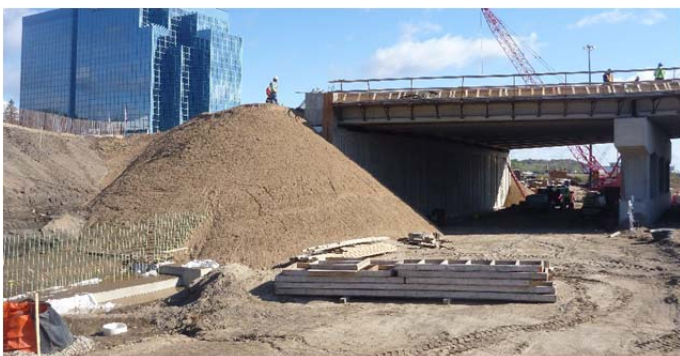
Fig.7. Adjacent retaining wall construction continues adjacent to the North Abutment, October 15, 2011.
