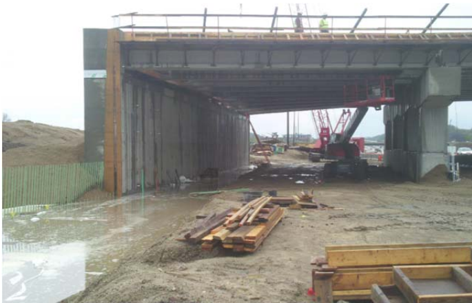
Fig. 6. North Abutment beams were placed October 12, 2011.
