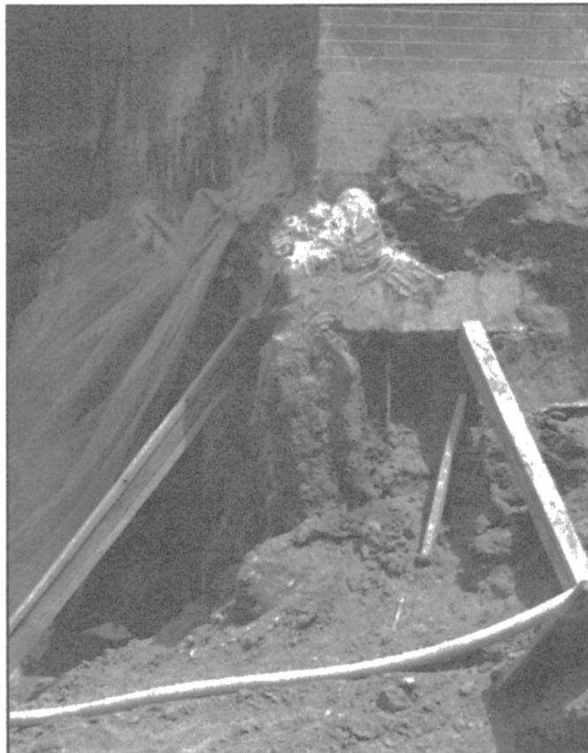
Pile #34 bracing is for personal protection, not structural support
