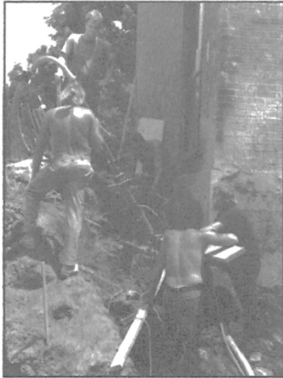
Grouting an anchor pile
