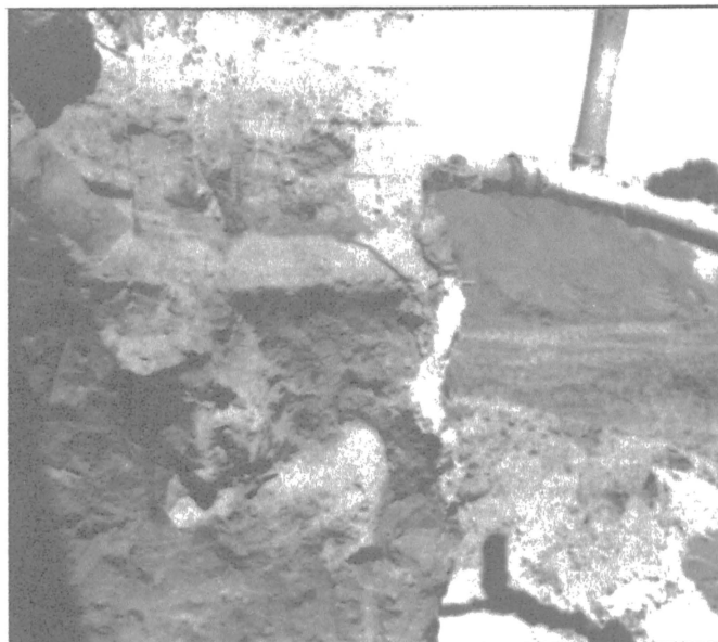
Final excavation before new footings
