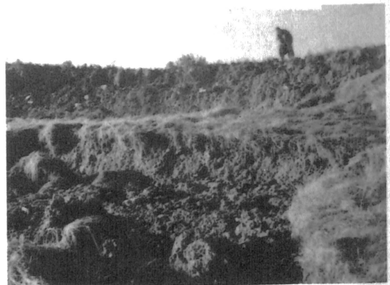
Fig. 2 Slide of downstream slope in 1948
