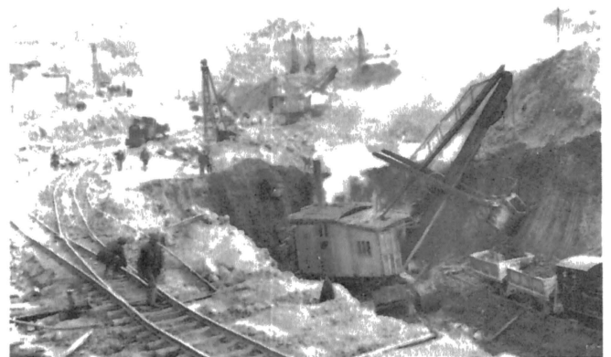
b) Steam shovel excavator
