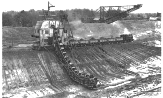
a) Multiple bucket excavating headrace canal
