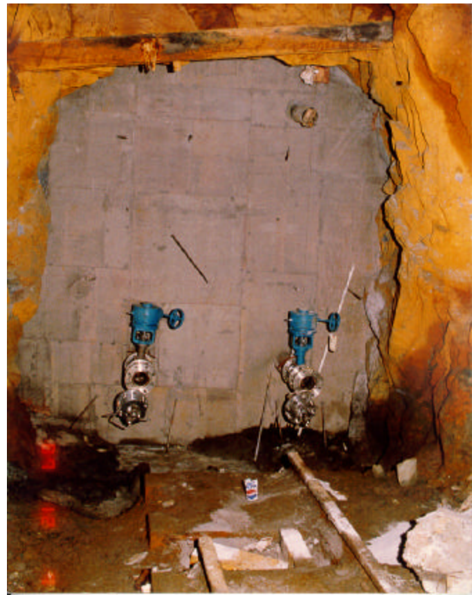
Photo 1. Seal after construction (December 1987).
