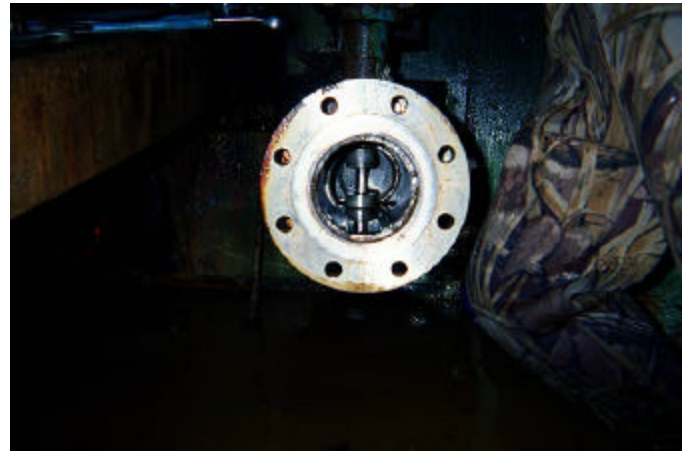
Photo 6. Interior of 4-inch control valve (June 13, 2001).
