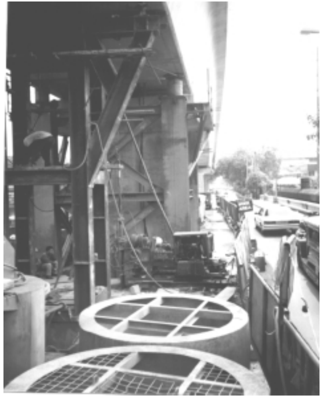
Fig. 7. Jet Grouting Equipment Layout
