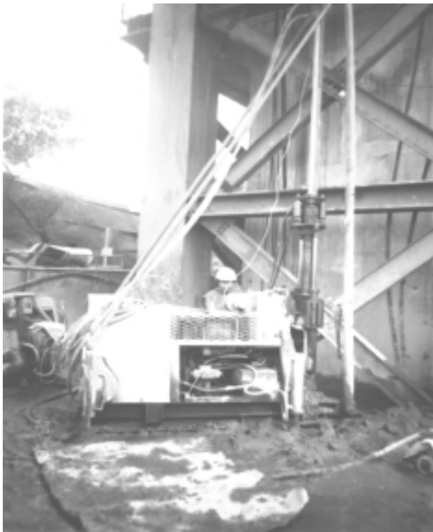
Fig. 6. Jet Grouting Machine set up under Pier
