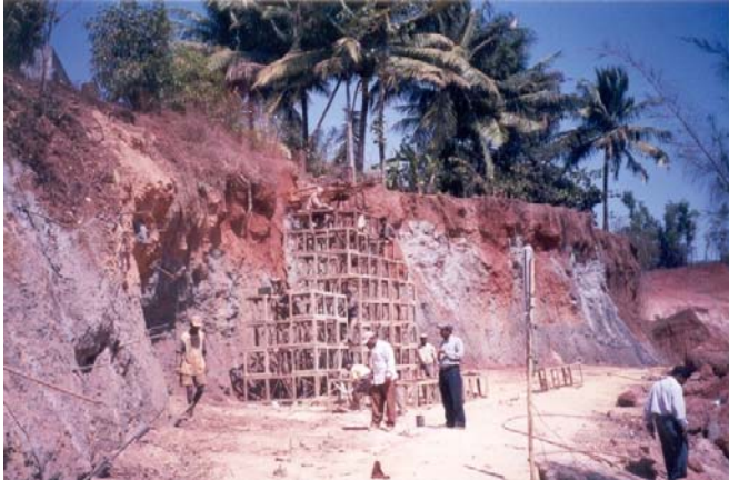
Fig. 4. Construction of Soil nail
