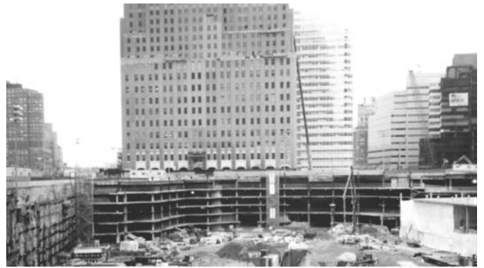
Fig. 12 Remnant basement structure at Vesey Street.
