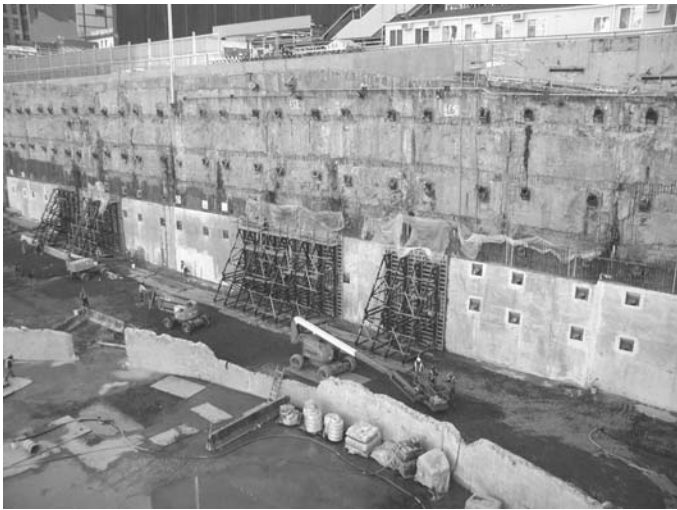
Figure 17 – Construction of liner wall at Liberty Street
