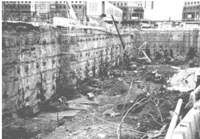
Fig.10 Tiebacks reinstalled at Liberty Street.
