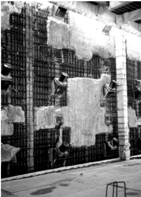
Fig. 18 Repairs of damaged slurry walls
