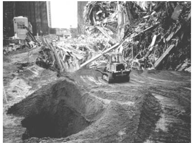
Fig. 6 Backfilling operations at Liberty Street.
