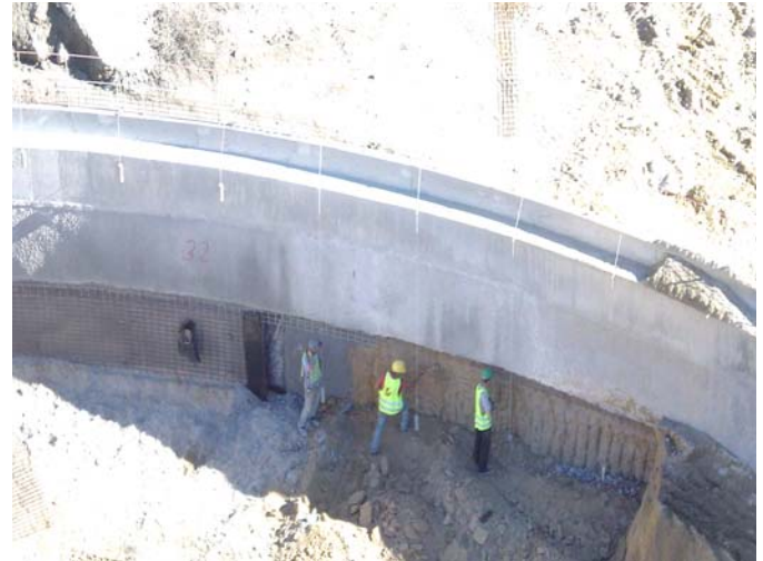
Fig. 4. Example of the excavation for a pane at Salgueiros Station
