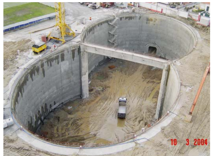
Fig. 5. Final excavation phase for Salgueiros Station
