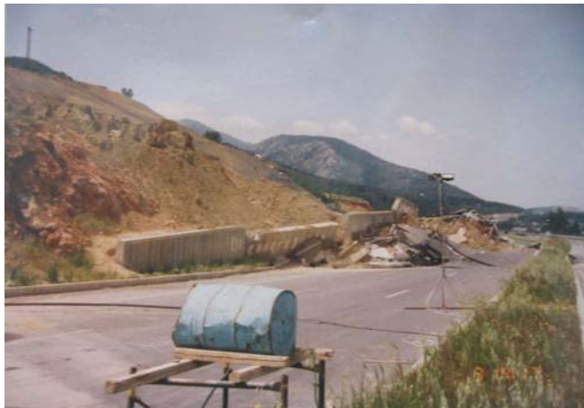
Fig. 2. Photo illustrating slide movement at its base (by Stamatopoulos)
