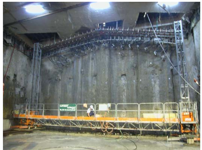
Fig. 22. Manifold system at the tunnel face and horizontal freeze-lances
