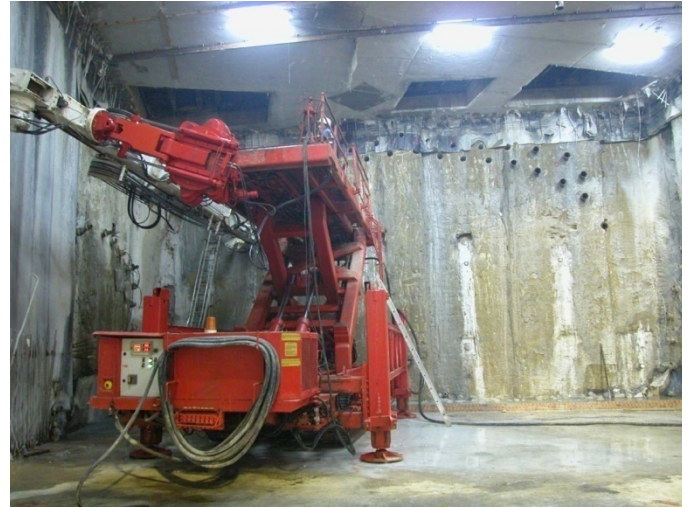
Fig. 21. Equipment during the drilling by HDD for horizontal freeze-lances installation.
