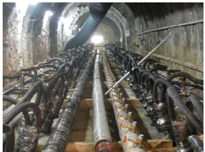
Fig. 23. Drift manifold system and inclined freeze-lances
