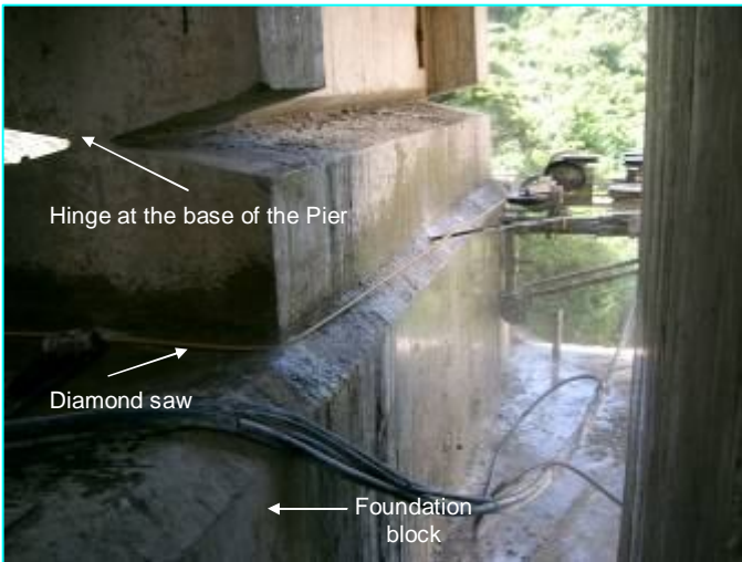
Fig. 17 a Diamond saw performing a cut at the base of Pier 9'
