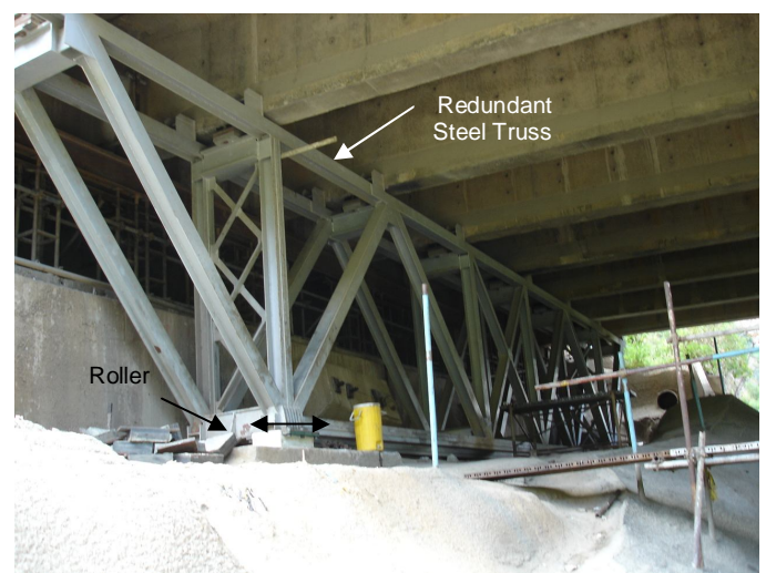
Fig. 14 Redundant truss at the Caracas Abutment
