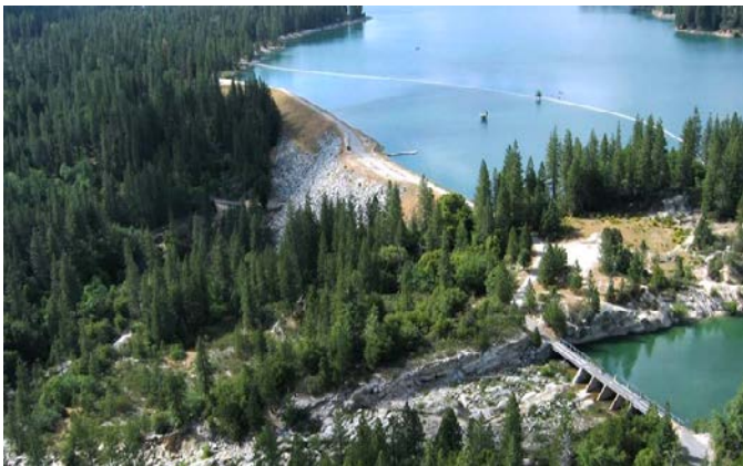
Fig. 1. Aerial View of Crane Valley Dam and Spillway.
