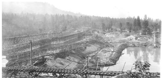
Fig. 3. Enlarged (1911) Dam Embankment.
