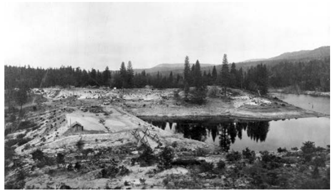
Fig. 2. Original (1901) Dam Embankment.
