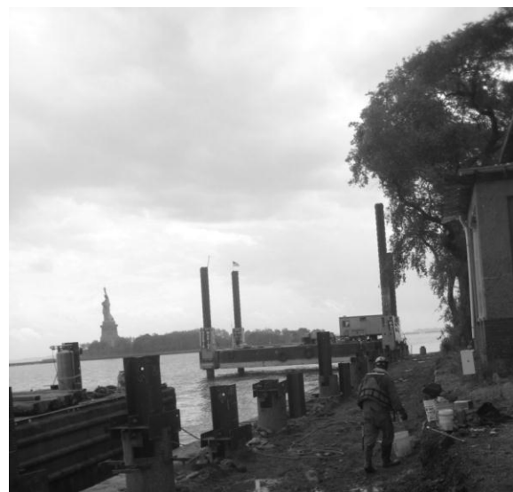
Fig 4. Typical driven piles and seismograph locations with respect to the buildings.
