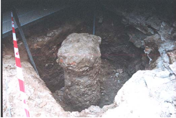
Fig. 6. Jet-grouting column.
