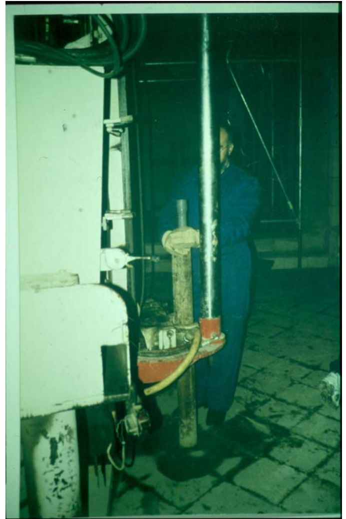
Fig. 2. Bore holes machine working inside the church
