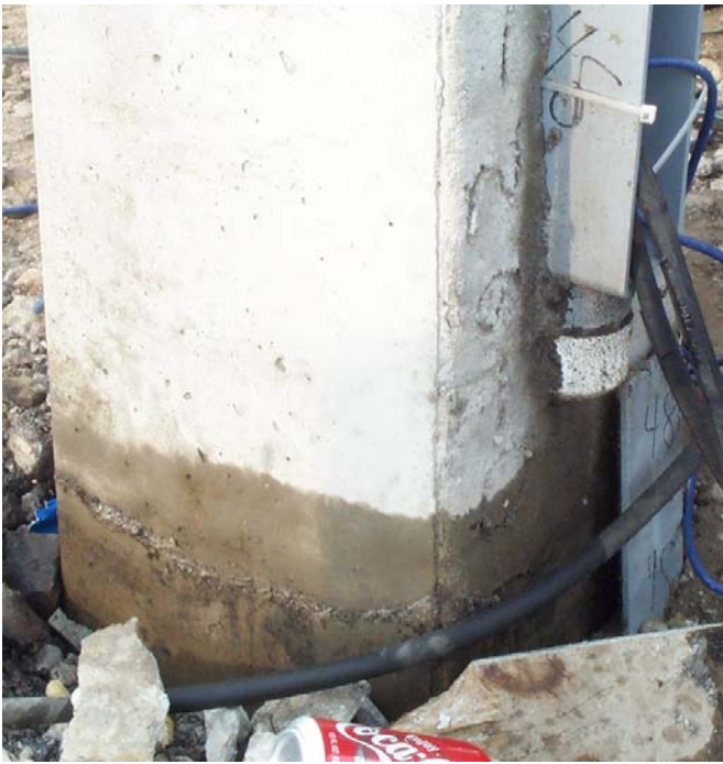
Figure 5. Pile pushed out of Ground during Osterberg Cell Test
