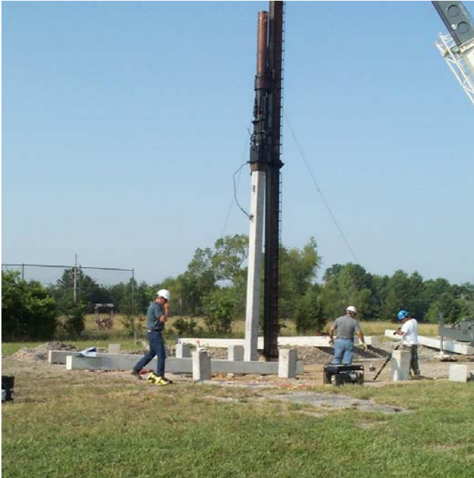
Figure 3. Pile installation in Progress
