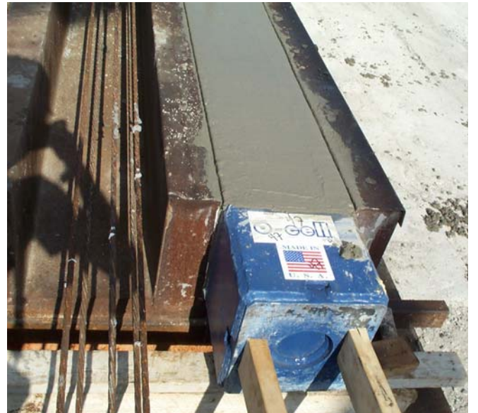
Figure 2. Construction of pile with O-Cell
