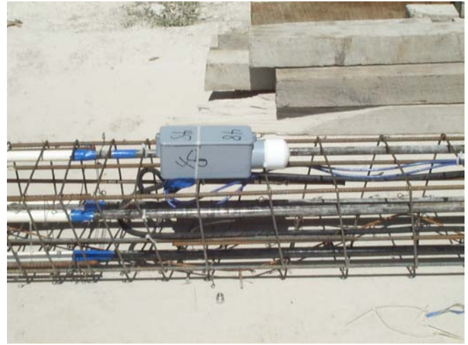
Figure 1. Instrumentation of the pile
