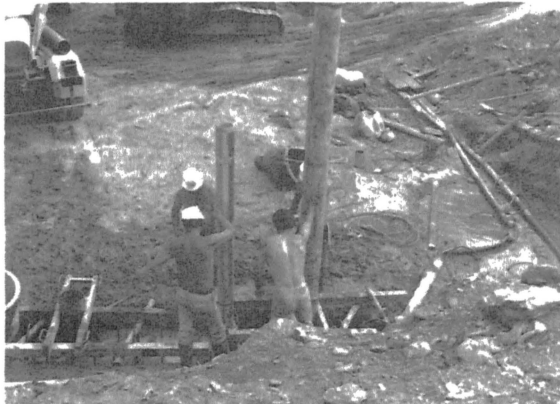
Fig 11: Preparation for Concreting for a Drainage Element
