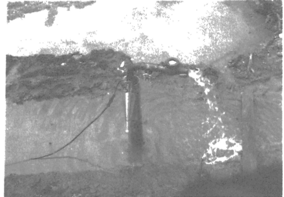
Fig 12: Pumped off Groundwater using a Drainage Element
