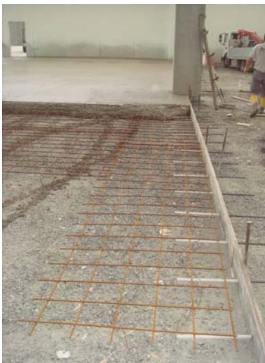
Figure 49. View of the industrial pavement during construction.
