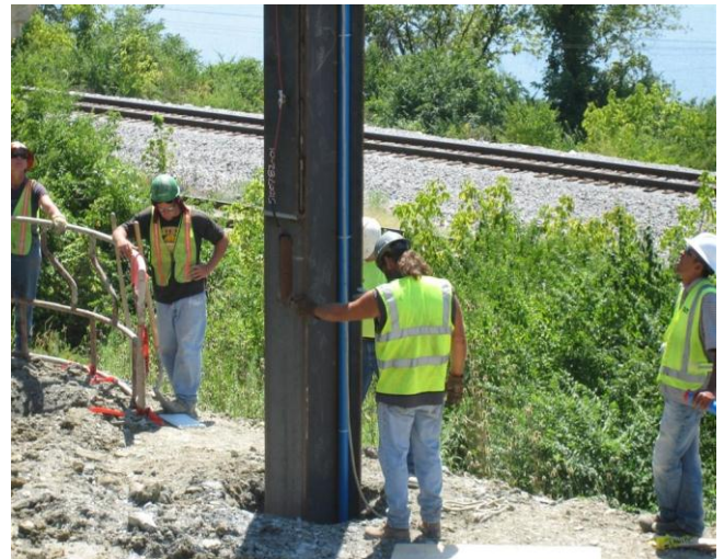
Fig. 10: Setting instrumented steel beam into shaft excavation.
