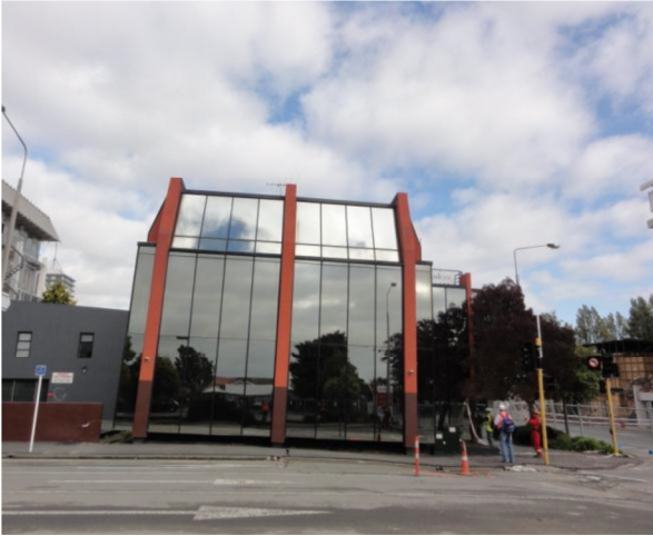
Figure 12. A three-story building subject to liquefaction-induced differential settlement and sliding (GEER, 2011)
