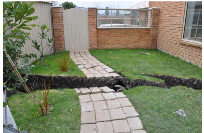
Figure 8a. Large ground cracks due to lateral spreading at Kokopu Pl (GEER, 2010b)
