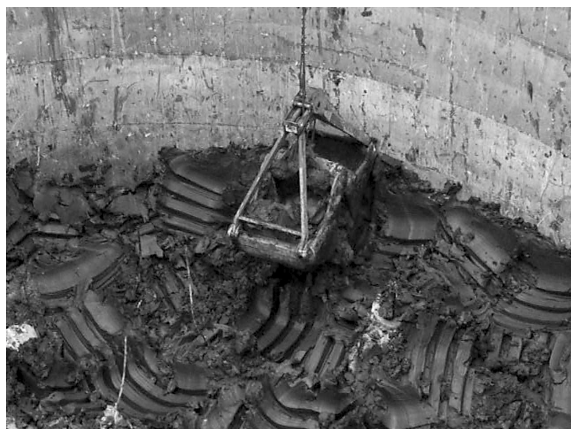
Fig. 6. Photo showing excavation inside caisson.
