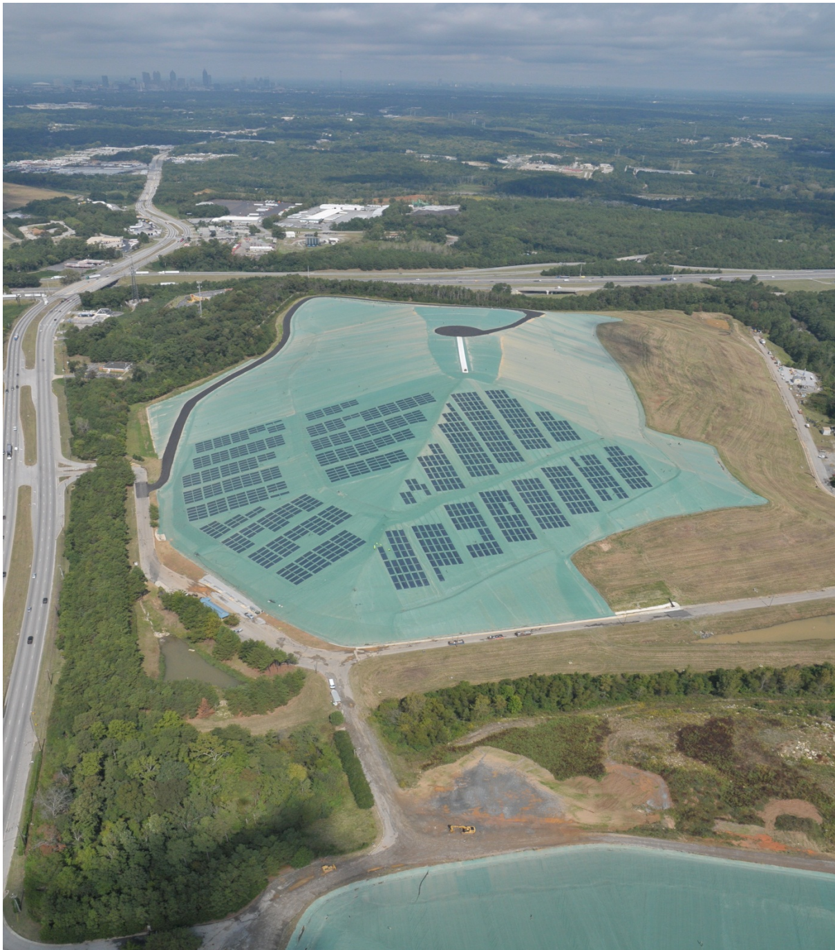
Figure 22 Solar Panels on Top of a Closed Landfill: Hickory Ridge Landfill 19
