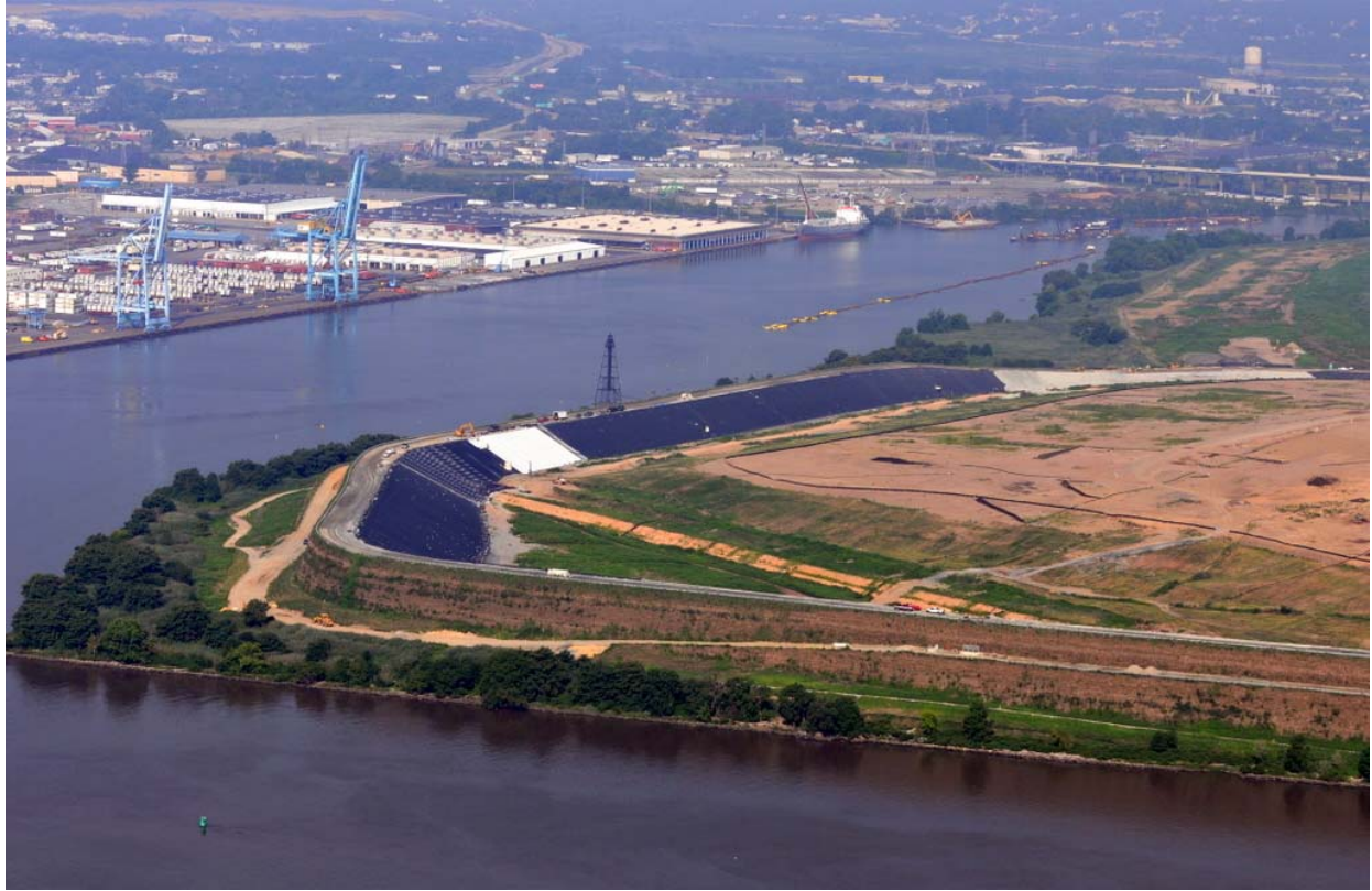
Figure 6 Landfill Liner Installation behind the MSE Berm (Geosyntec, 2012)
