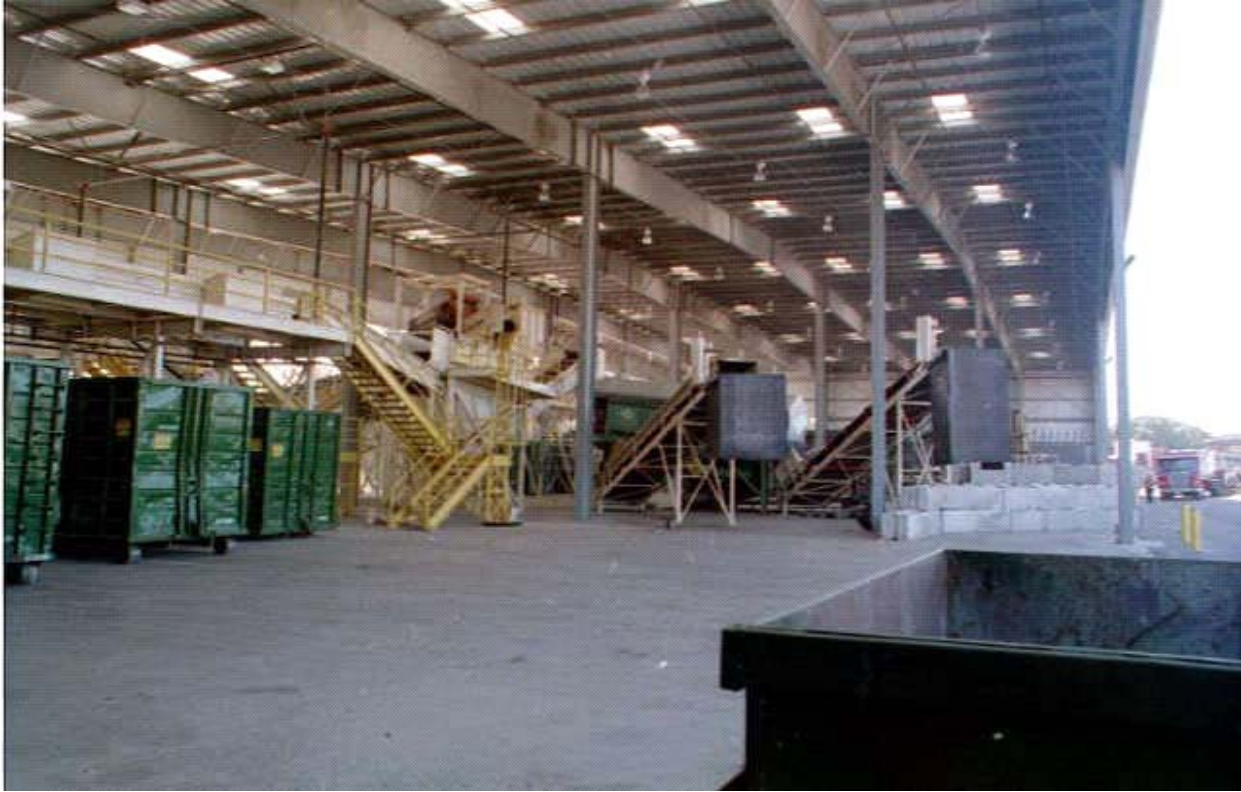
Figure 19 shows a photo of the Inside of the Completed building (Sharma, 2012)
