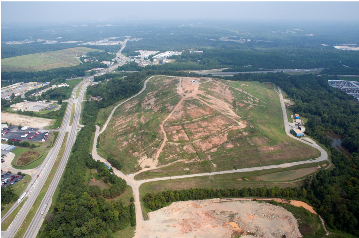
Figure 21 Hickory Ridge Landfill Prior to Installation of Solar Panels 18
