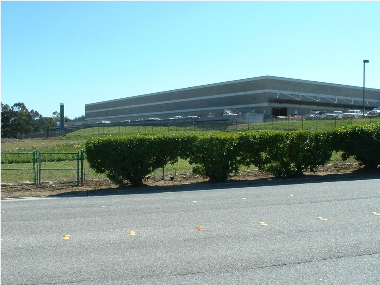
Figure 18 A View of the Completed Commercial Building with Gas Flare System Shown on the Left (Sharma, 2012)
