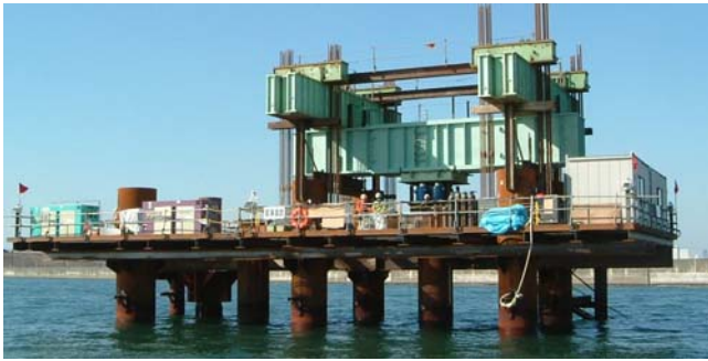
Fig. 9. View of static axial compressive load test.
