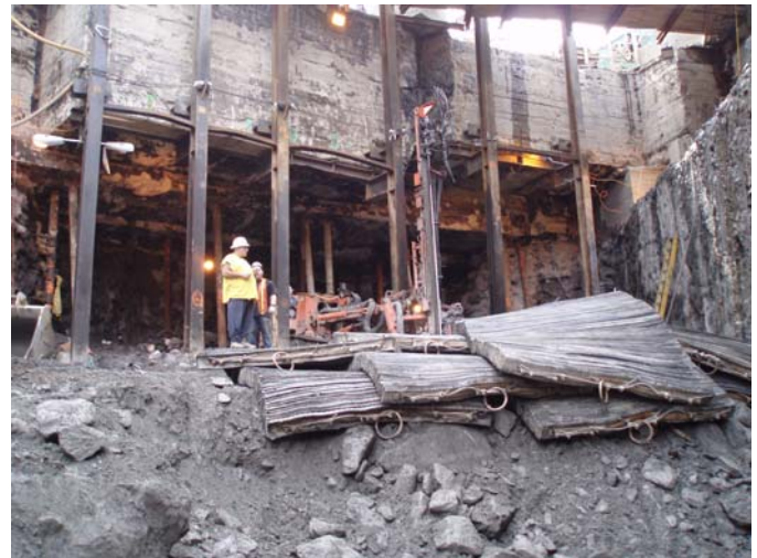
Fig. 3. Blasting beneath subway, between underpinning piles
